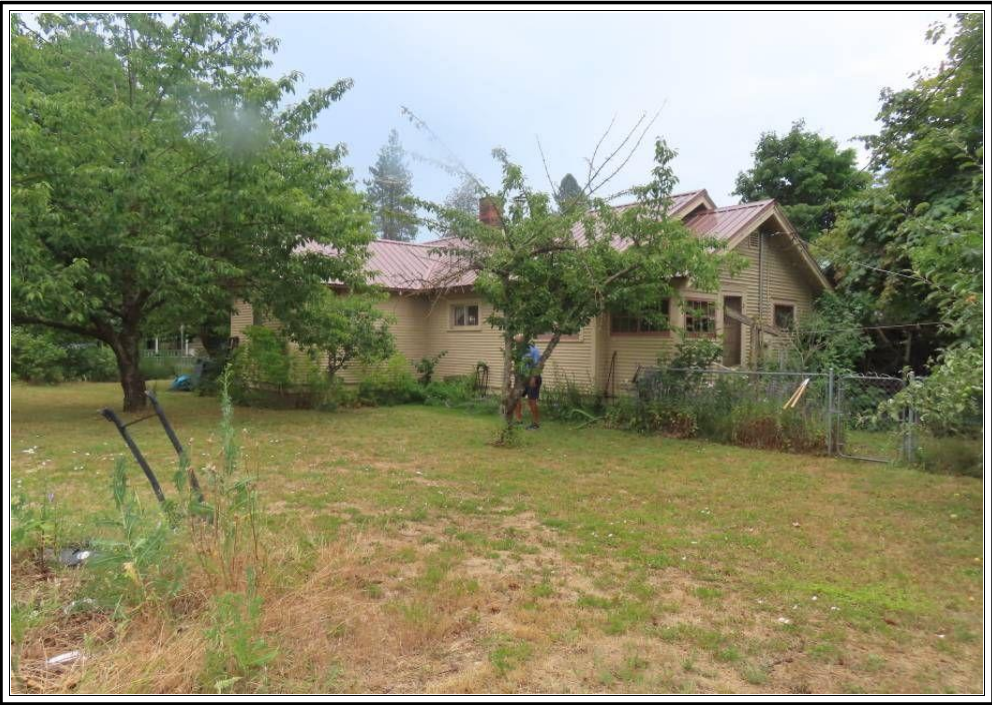
REAR OF SUBJECT PROPERTY
